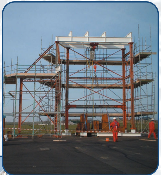
25 tons deflecting test
